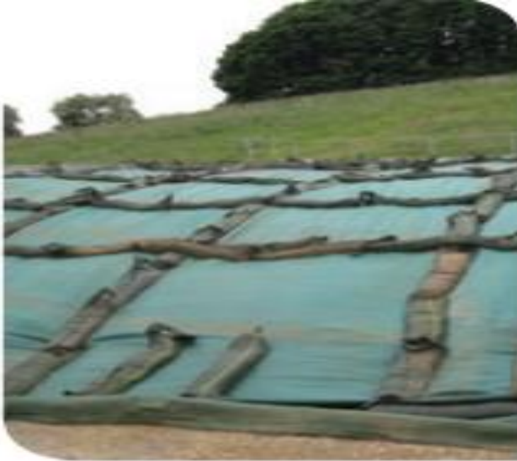
Figure 1.3 Sealing stack with bags
